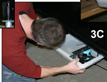
Sliding Condensate Pump Pan under case
