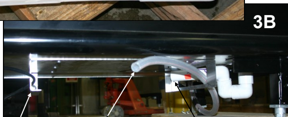
Condensate Pump Pan Support Bracket (one at either side) Condensate Pump Hose Drain Pipe (to be positioned over condensate pump pan)
